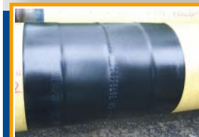
Heat- shrinkable sleeves
