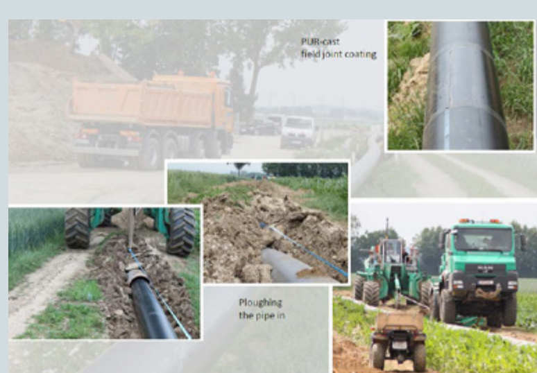
Figure 15: The coating combination of polyethylene and polyamide in the plough laying procedure
