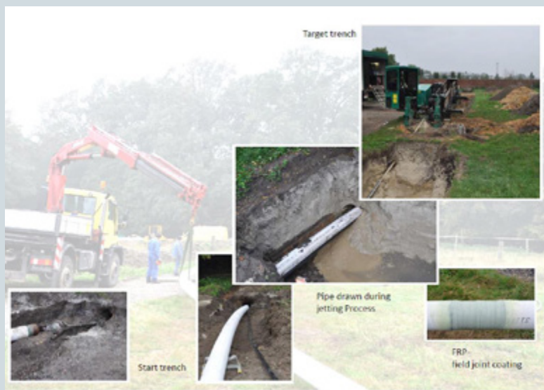
Figure 16: The coating combination of polyethylene and polypropylene in the jetting process
