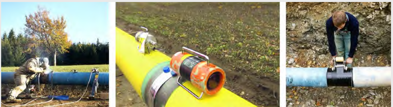
Figure 1: Welding, testing and field coating
